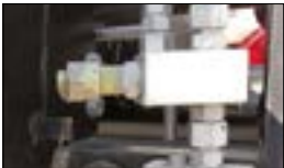
End of cable/ hook upper position automatic movement stop
